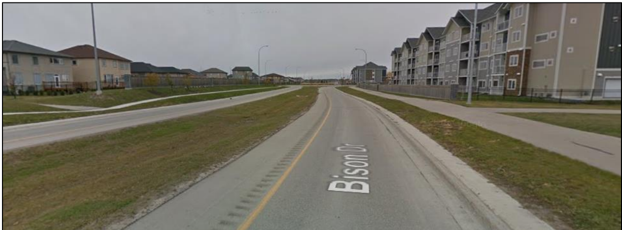
Photo 1: Image of Crossing Location Looking East (source: Google Streetview)
