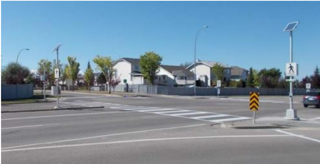
Photo 5: Typical RRFB Pedestrian Crossing Installation on a Four Lane Divided Roadway.
