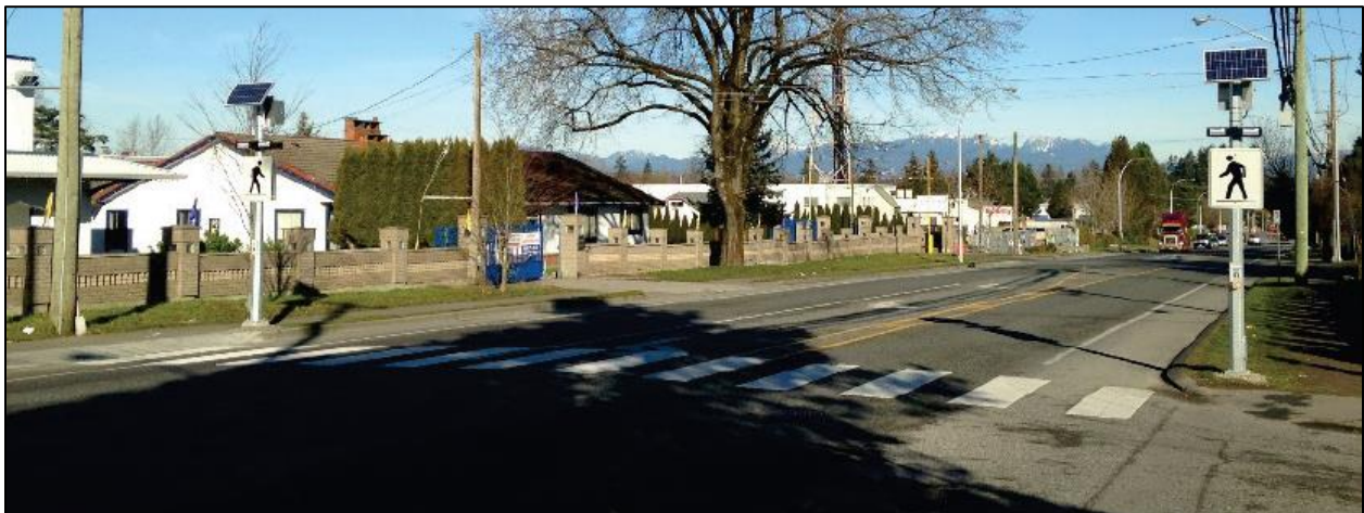
Photo 4: Rectangular Rapid Flashing Beacon (RRFB) Installation (source TAC)
